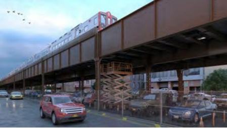
Park Avenue Viaduct Replacement Project:
